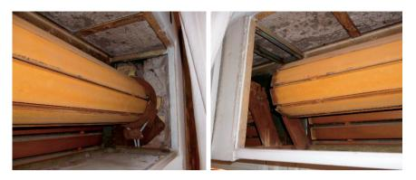
Figure 8 – Detail of the box and roll-down blinds
