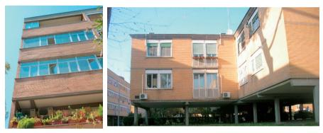
Figure 4 - Closed off balconies with different types of windows (left) and the addition of air conditioners
